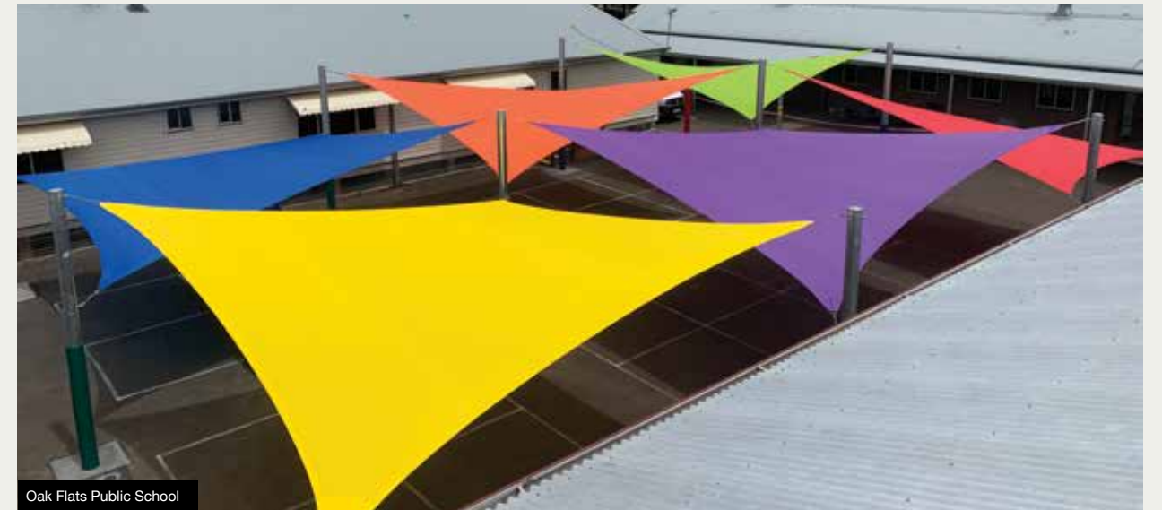
Oak Flats Public School
